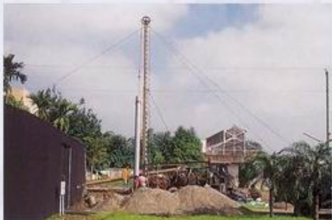
▲ 水井工程 Well drilling engineering
