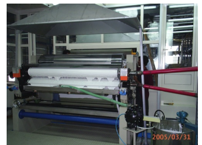
Coil Coating Line Equipment
