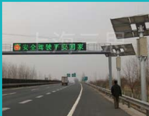
Variable Message Signs for Highway
